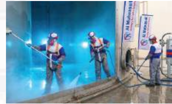
Water Tank Cleaning
